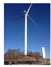
Varian Semiconductor, a private technology supply company, recently constructed a 2.5 MW turbine adjacent to it's headquarters in Gloucester, MA. The 100 meter (328 foot) turbine, with a 100 meter blade diameter, is the largest in the northeast and will supply about one third of the companies power. Construction site plans were prepared by Atlantic Design Engineers, addressing site access, turbine component
